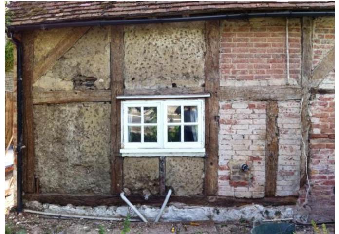
The original facing exposed, the left hand side showing the wattle, the right hand, the brick infill
