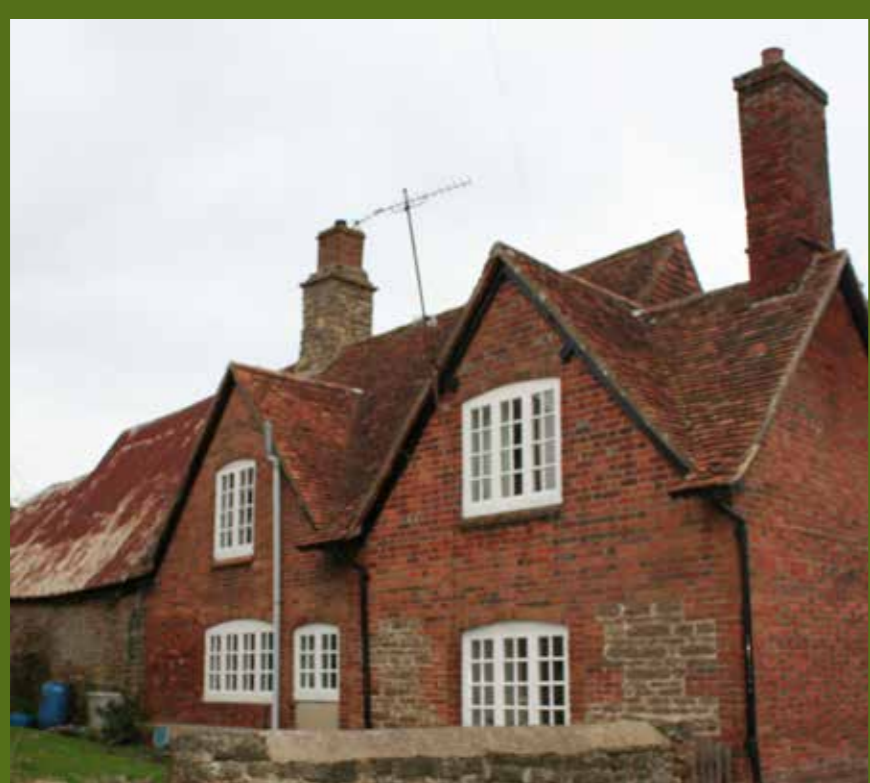
1 Varying roof pitches and chimneys create distinctive roofscapes
