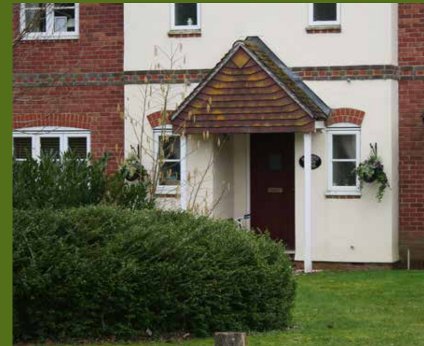
6 Landscaping helps soften the built form
