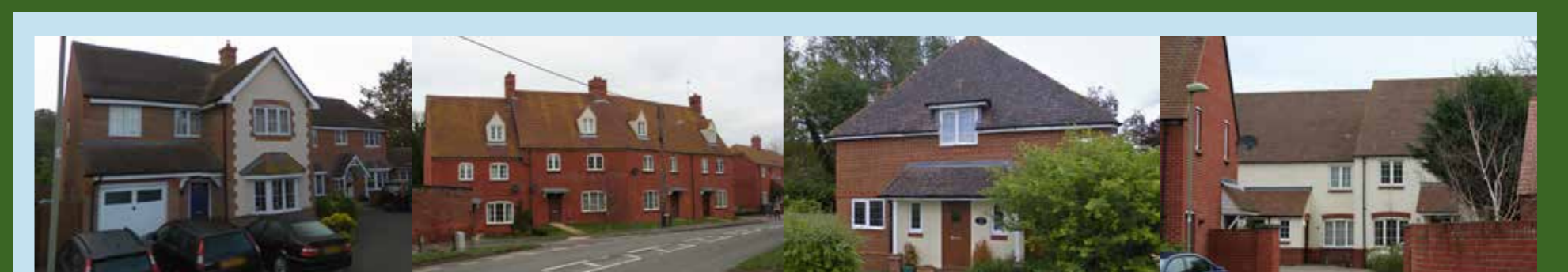
LESPORE CLOSE - RED BRICK, RENDER AND CONTRASTING SURROUNDS/QUOINS ANIMATE THE BUILDING ELEVATION STEVENTON ROAD - A STRONG BUILDING LINE OFFERS CONSTANT SURVEILLANCE TO THE STREET AND INCREASES LEGIBILITY ABINGDON ROAD - FULL HIPPED ROOFS AND A DORMER WINDOW CREATES A DISTINCTIVE ROOFSCAPE BARN COURT - A MIX OF RED BRICK AND RENDER CREATE INTERESTING STREET SCENES
