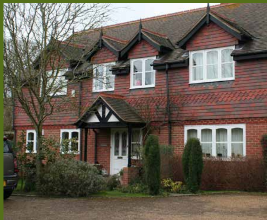
5 Feature gablets break up the roofscape
