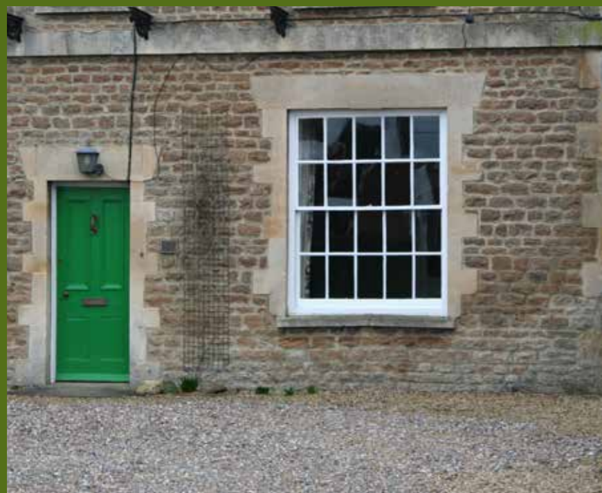
4 Stone surrounds to door and windows
