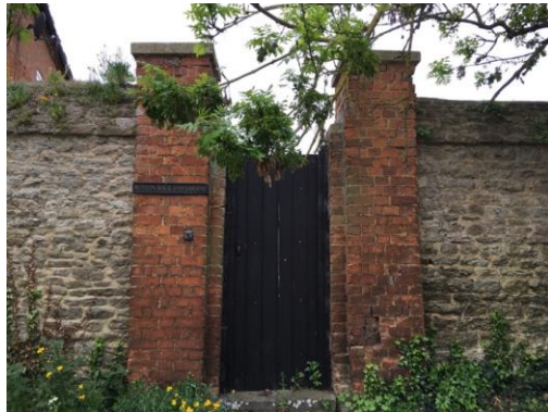
Stone boundary wall with brick gate piers
