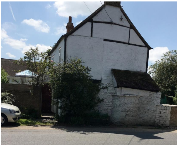
Figure 28 Walnut Tree Cottage showing timber-framed gable and bread oven
