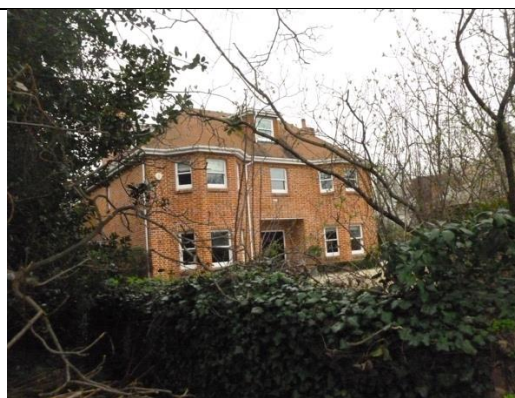
Bradfield House, High Street – house, 19thc, two-and-a-half storeys, double fronted and double pile. Brick in Flemish bond with plain tile roof. Symmetrical bays either side of centre.
