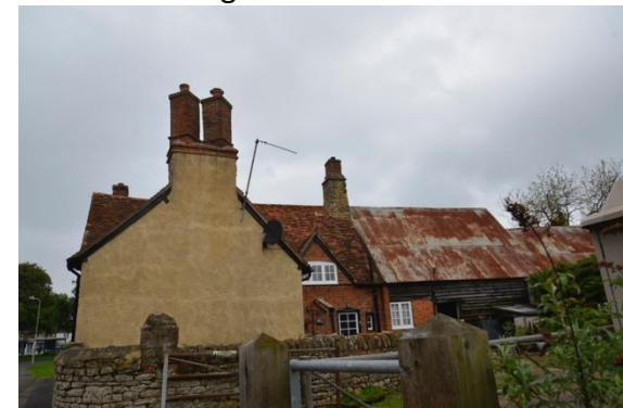
Timber framing with brick infill
