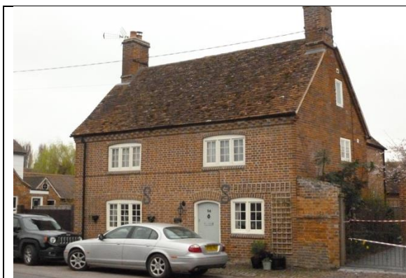
Carpenters Cottage, 54 High Street – two-and-a-half storey brick cottage with plain tile roof. Flemish bond. Maybe late 17thc in origin. Off centre door, casements windows
