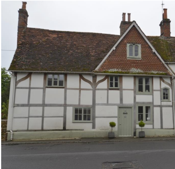
Figure 25 Attractive seventeenth-century timber framing at 44 High Street
