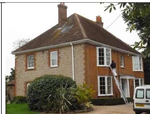
Elm Close, 71 High Street – house, 19thc two-and-a-half storey, double fronted and double pile. Brick front, in Flemish bond, with coursed rubble flank wall. Bays either side of entrance with 4 over 4 sashes with pilasters. Central classical portico with slender columns.
