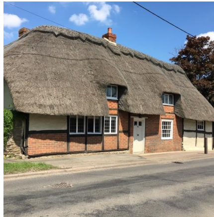
Cruck framing (exposed on gable) with thatched roof
