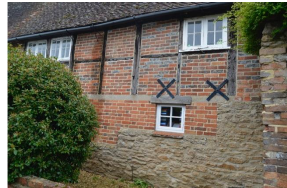
Timber framing with brick infill
