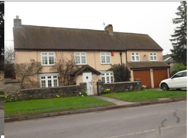
Yew Tree Cottage, High Street – House, two storey, 3-unit. Painted render with plain tile roof. End stacks. Central porch. 20thc windows
