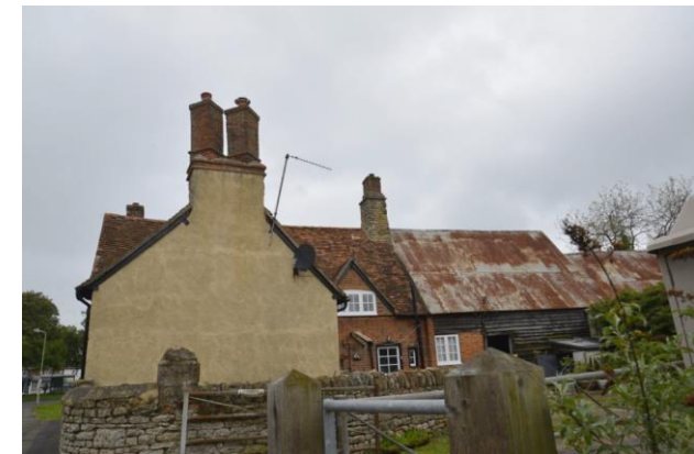
Figure 31 gravel Lane with attached barn and outbuilding
