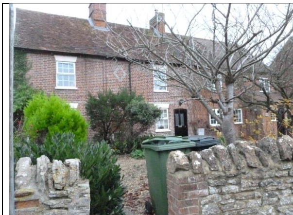
Church Lane – cottages – late 18thc or early 19thc, two storey. Flemish bond brickwork with plain tile roof. Ridge stacks and decorative motif in centre of terrace
