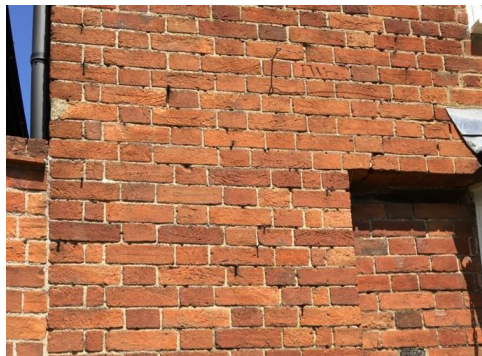
Flemish bond brickwork
