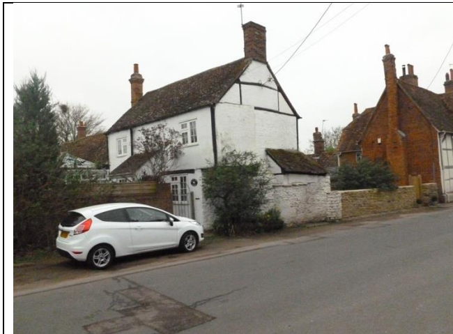
Walnut Tree Cottage, High Street – house, two-storey, painted brick with plain tile roof. Flank wall facing onto road has remnants of slender timber framing in gable. Projecting bread over.
