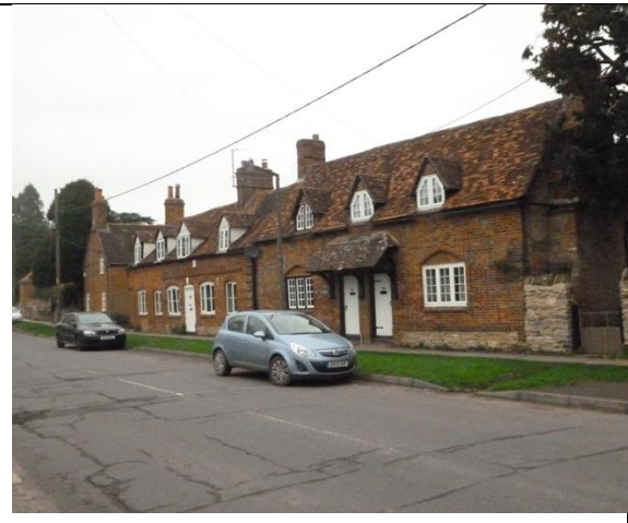
27-29 High Street - cottages, one-and-a-half storeys. Brick with plain tile roof. Casements windows to ground floor, dormer to roof space
