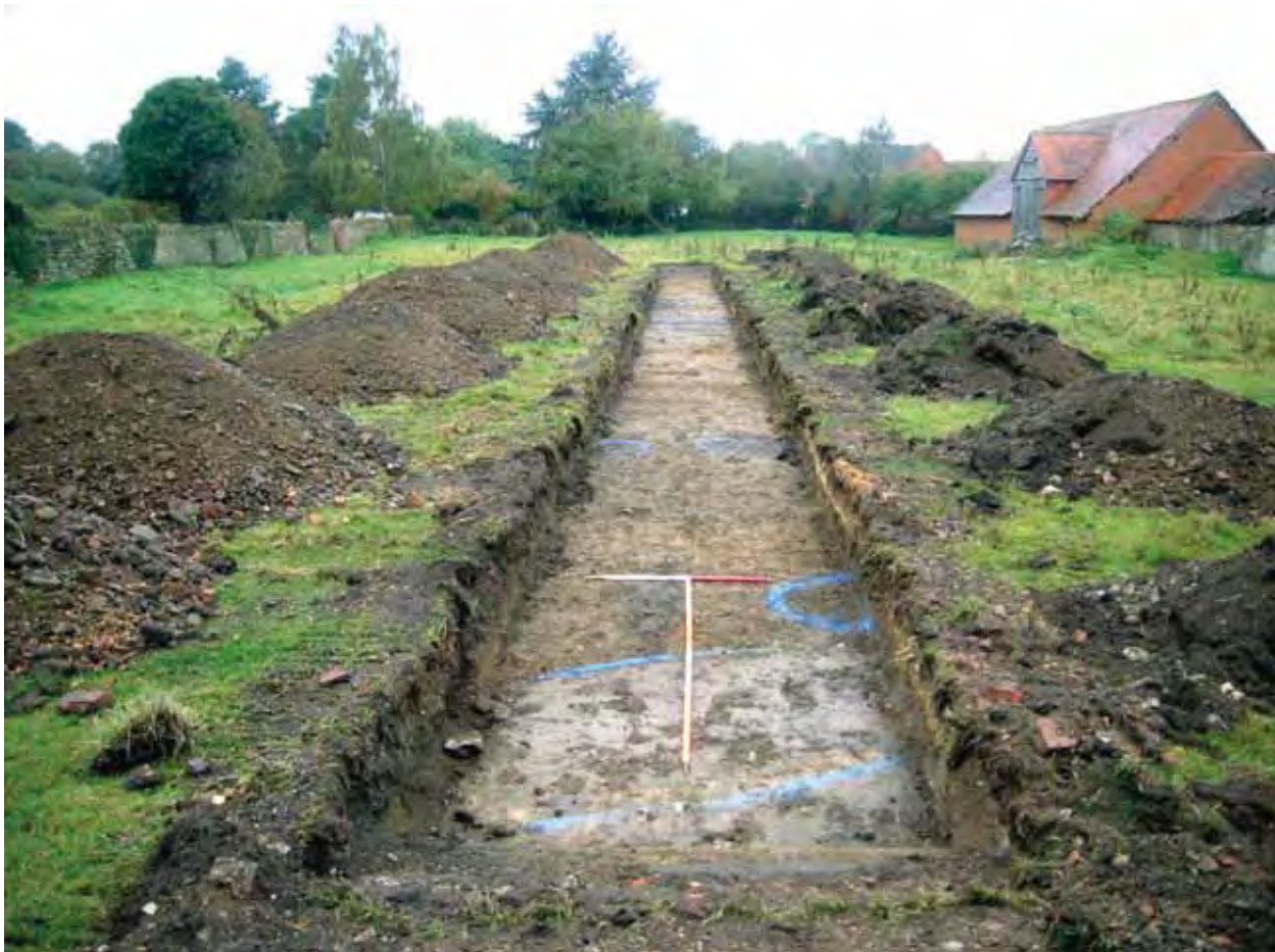
Plate 2: Trench 7, view to the west
