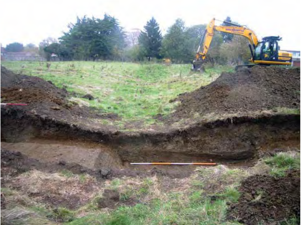
Plate 5: Ditches 905 and 907, section 901, view to the north
