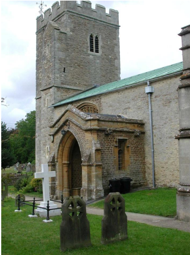
St Peter's Church Tower, Church Lane, Drayton
