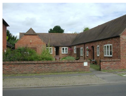
Alms Houses, High Street, Drayton
